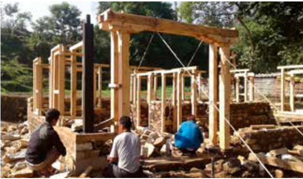
Banepa: The city wants to preserve traditional building methods.
