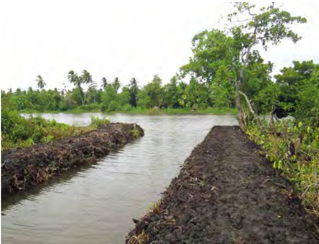
Left: Rehabilitated drainage channel.
