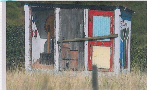
IN DIRE STRAITS: Buloghe Farm School, situated just outside East London, is one such school that had to make do without proper toilet facilities. The school, which has 250 pupils enrolled, made use of a single pit latrine while other pupils were forced to relieve themselves in the bushes Picture: MARK ANDREWS
