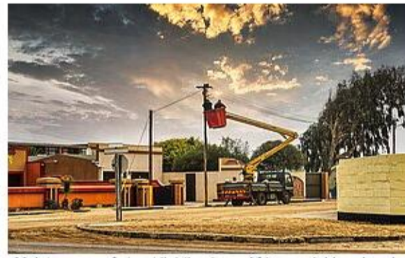
Maintenance of street lighting in an African neighbourhood Photo: Lucian Coman | Dreamstime.com
