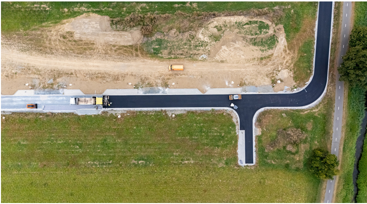
Construction of new roads for urban infrastructure development. Photo: Eduard Goricev, shutterstock
