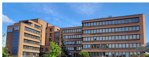
Interim use prevents damage until construction work begins on the renovation of the future town hall in Regensburg © Stadt Regensburg
